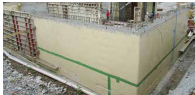
Open excavation with SikaProof® A, after removing the formwork the anchor penetrations has to be sealed.
