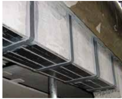
BEAM STRENGTHENING
