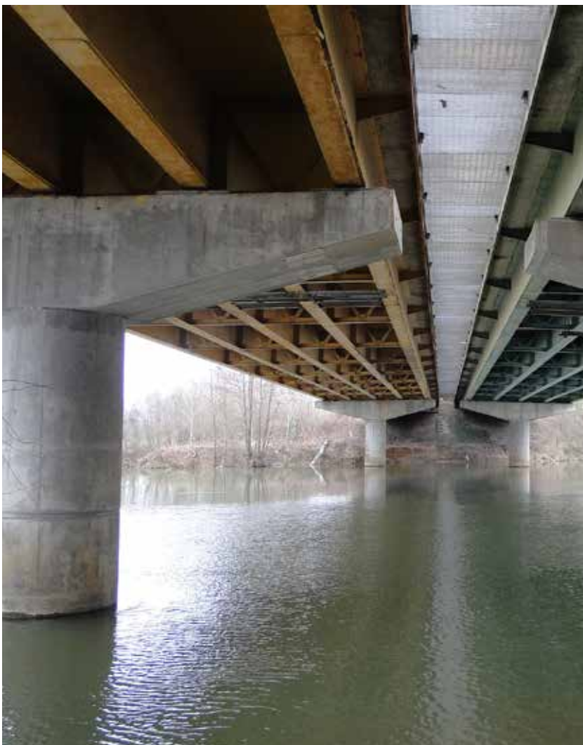
Two layers of Sika CarboDur®
