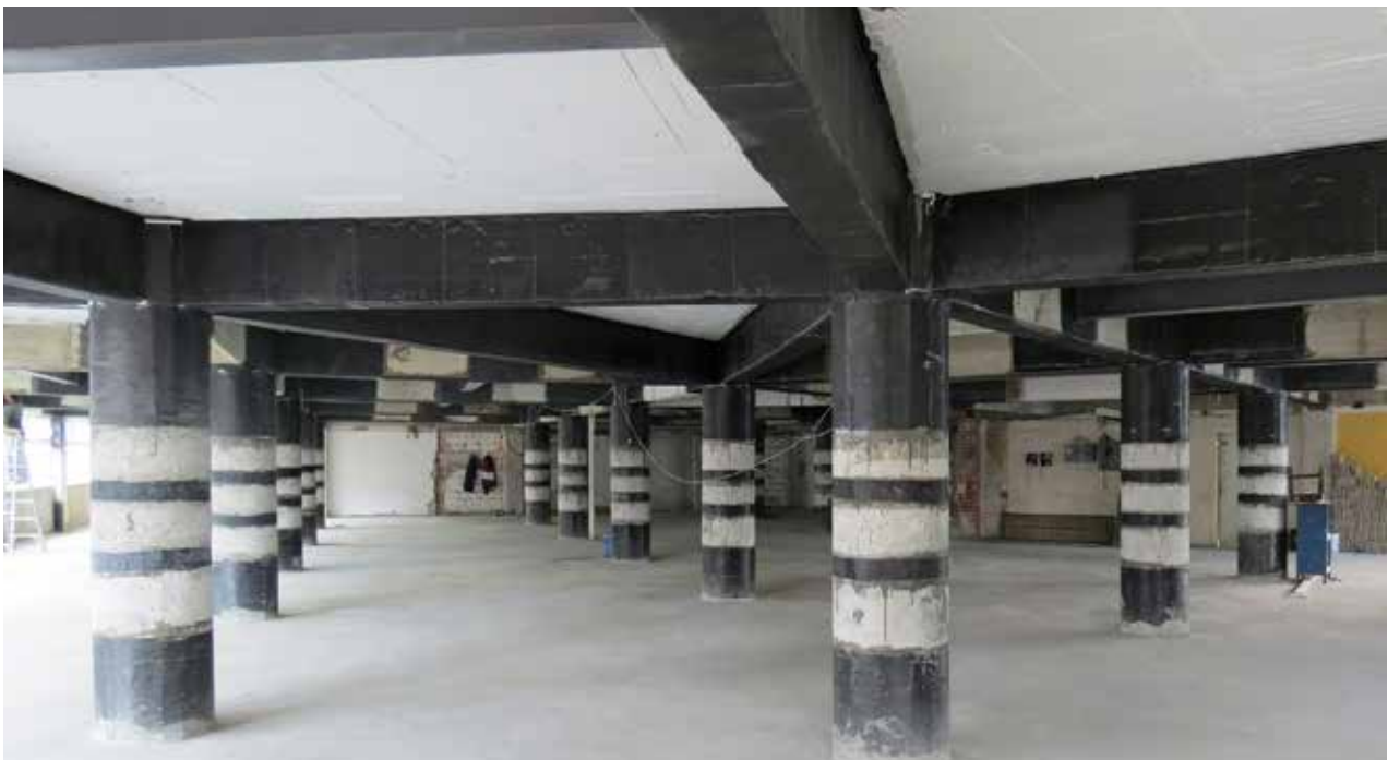
Beams and columns strengthened with SikaWrap®
