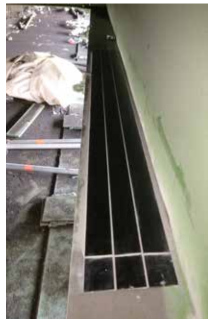
Two layers of Sika CarboDur®
