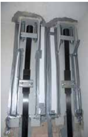
Anchorage of Sika CarboStress System
