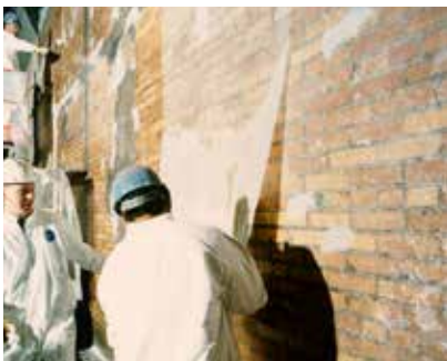
SEISMIC UPGRADING /EARTHQUAKE DAMAGE REPAIR
