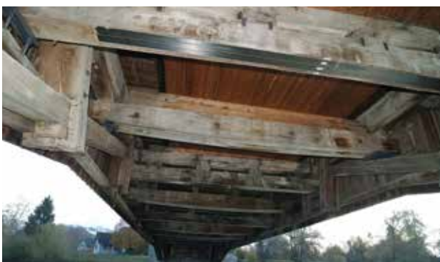
CarboDur® strengthened crossbeam
