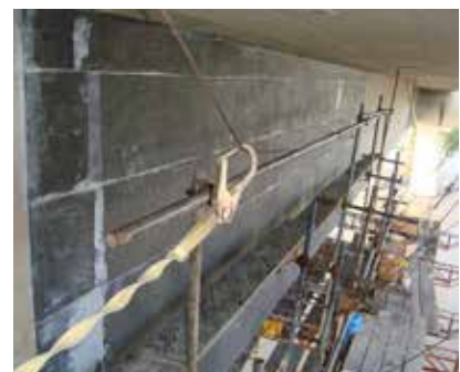
Strengthening with SikaWrap®
