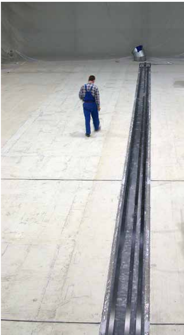
The longest post-tensioned CFRP-plates ever installed
