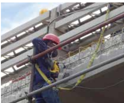
Substrate preparation
