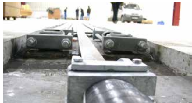
Base channel with post-tensioned CFRP plates
