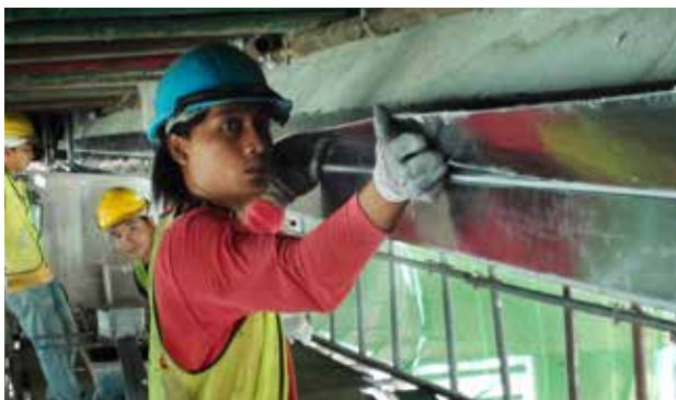
Installation CarboDur®
