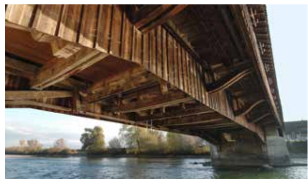
Bottom view of strengthening system
