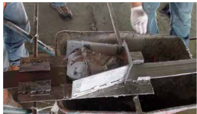
Coating of CarboDur® plates with Sikagard®
