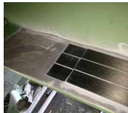
Two layers of Sika CarboDur®
