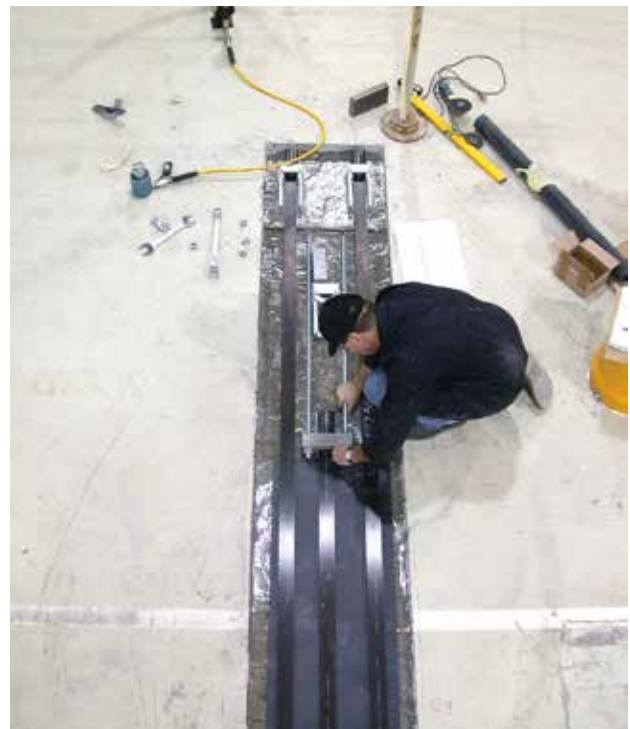
Plate and end-anchorage
