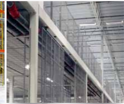
Mezzanines Partitioning mesh walls on a mezzanine protect both materials and people from falling objects.
