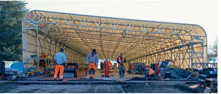
The Keder Roof XL is a lightweight, but very sturdy weather protection roof for great spans up to 30 m.
