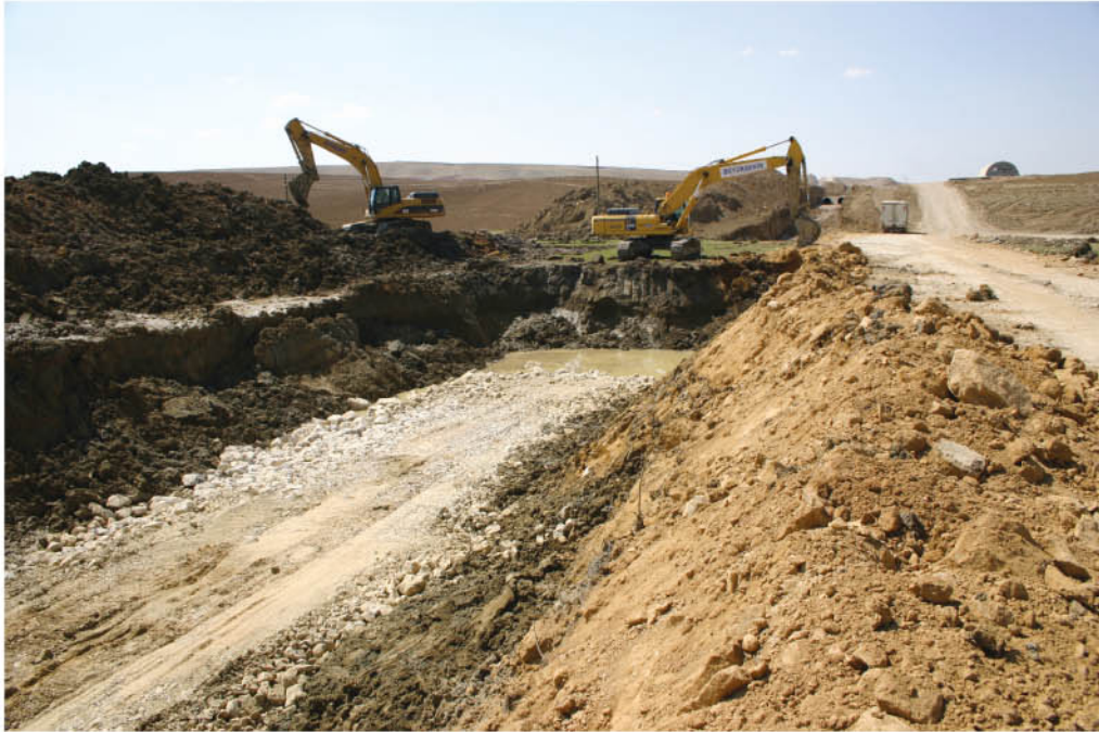
Trench ground stabilization works (Foundation)
