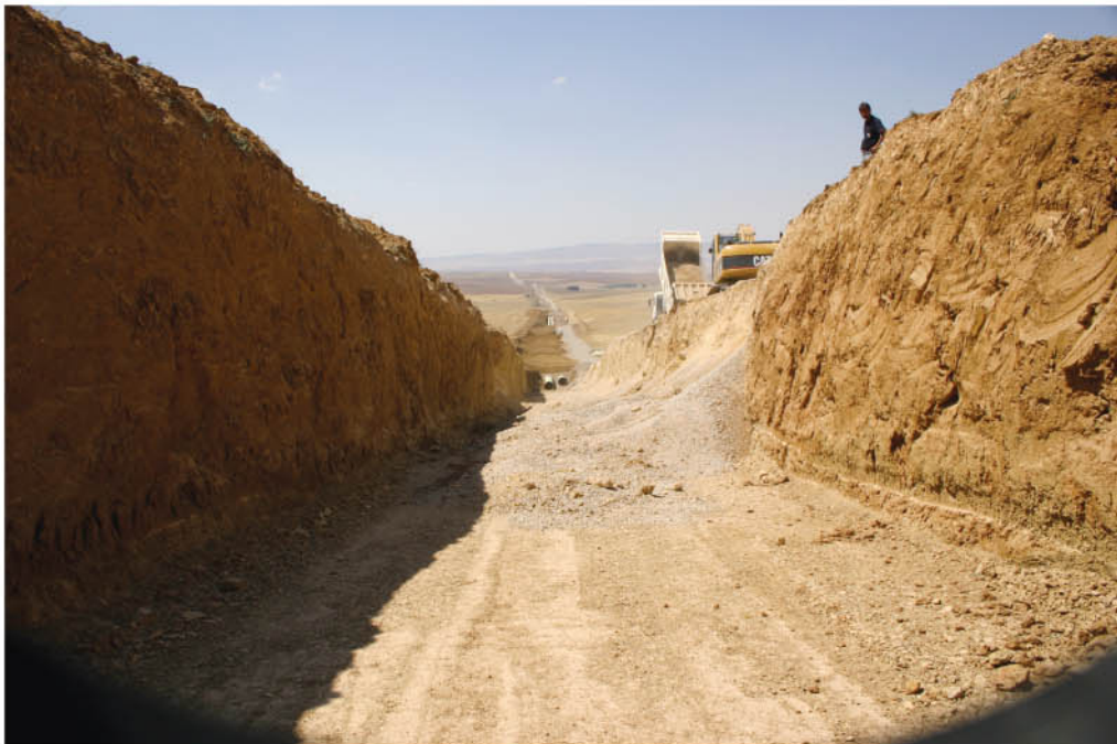
Bedding after ground stabilization
