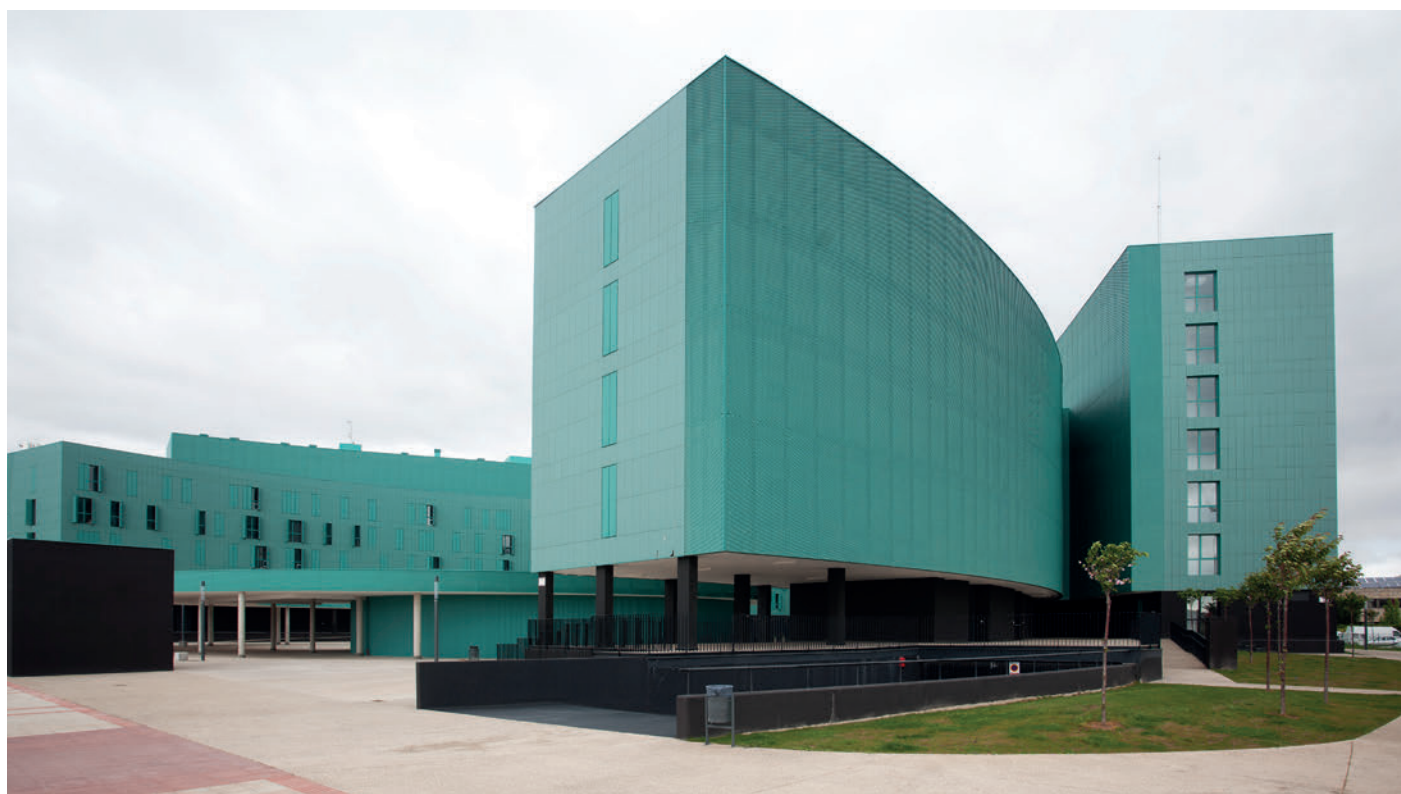
tempio®[projects] Dolcestone by Toyo Ito. Logroño, Spain.
